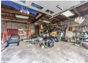
Insulated automatic garage door, concrete floor
